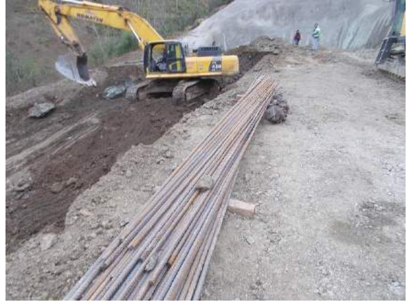
Picture 26 Slope cutting
