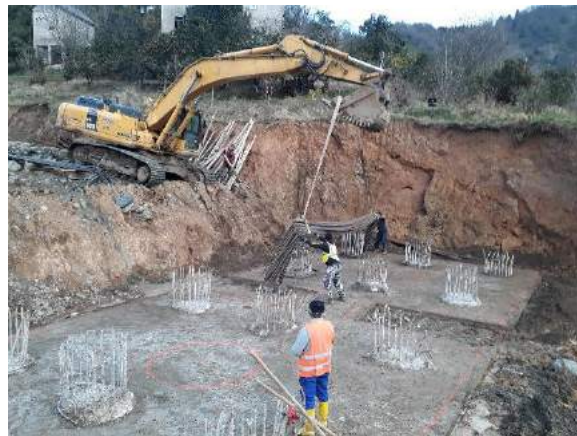
Picture 18 Pile foundations
